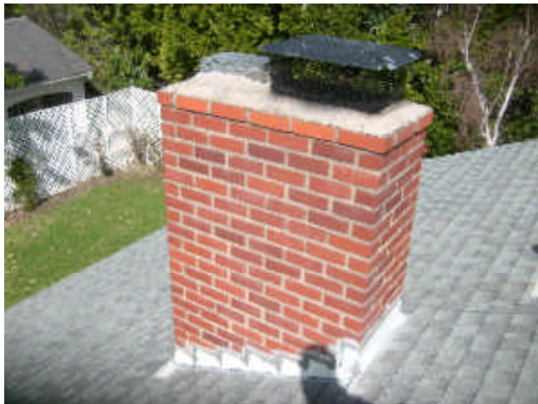
The chimney is made of brick.
