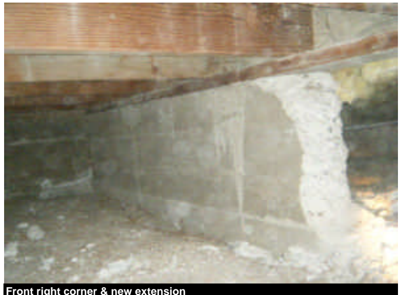
Front right corner & new extension
