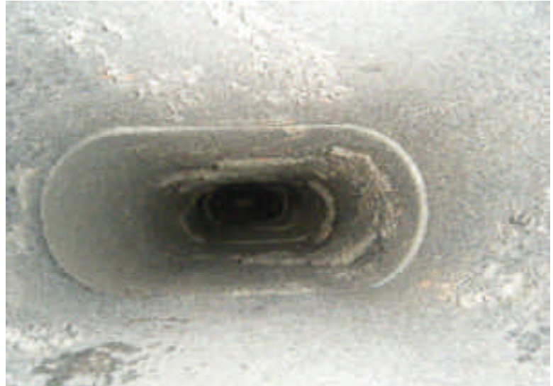
Looking down flue from roof.
