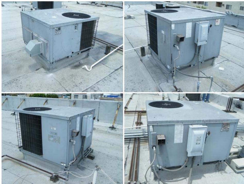
For the 2nd floor, there are 8 units, in similar condition.
