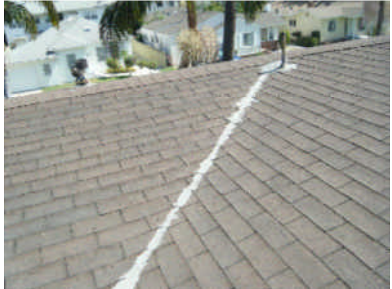
Excess caulking is used in the valleys in the front.
