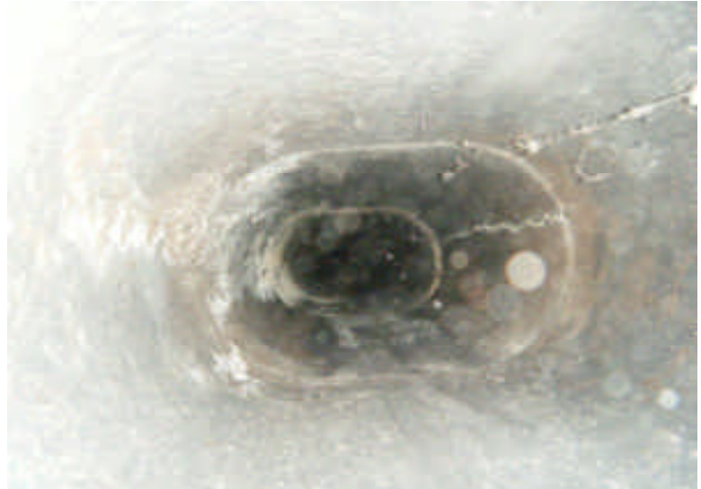
Looking down the flue
