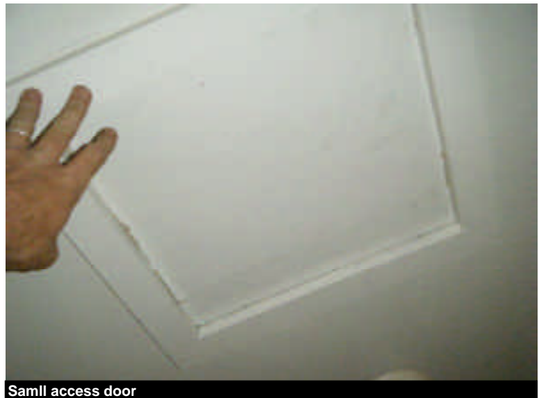
Small access door
