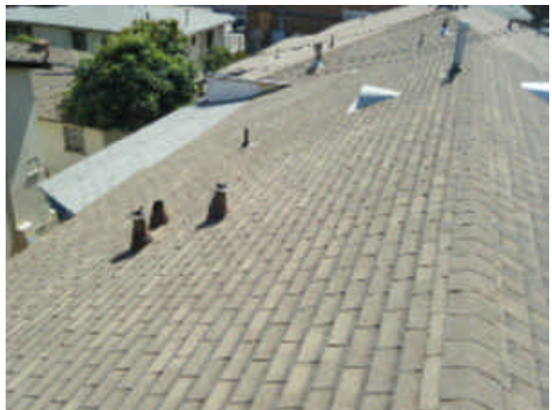
Note: The back building roof appeared generally serviceable with
