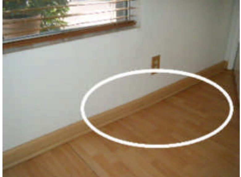
Not Acceptable, there are areas cupping and bowing pergo type flooring along the planter area especially near the front door.
