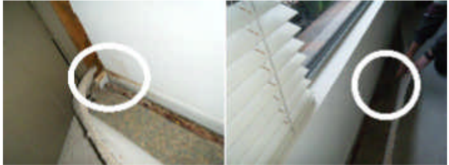
Not Acceptable. water stains and intrusion is found near the edge of the exterior planter and in the middle area.
