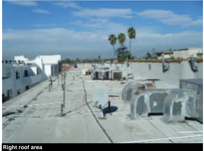
Right roof area
