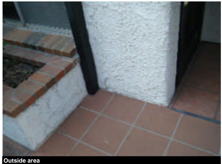
Not Acceptable. water stains and intrusion is found near the edge of the exterior planter and in the middle area.
