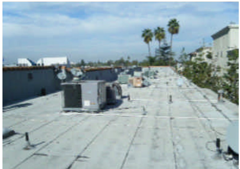
Left roof area
